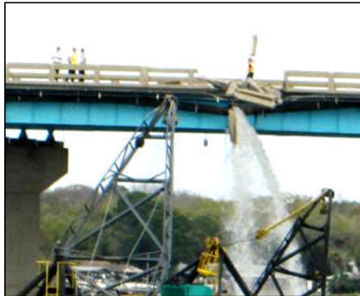
Brooks Bridge after it was struck by a barge carrying a crane at 3:15 pm on Wednesday, March 20. The water fall is from a broken water line.
